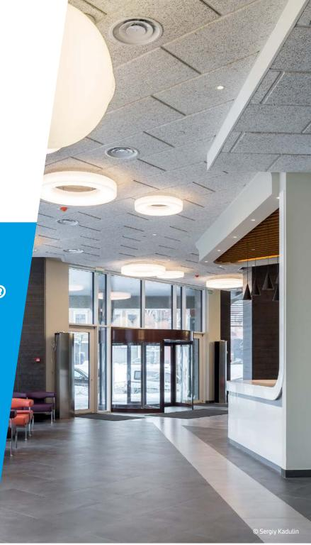
HERADESIGN® Macro is a acoustic ceiling and wall panel made from single layer, magnesite bonded wood wool (fibre width 3mm).
