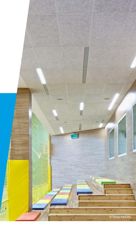
Homogeneous wood wool panels with acoustic fleece, higher sound absorption with the same panel thickness.
